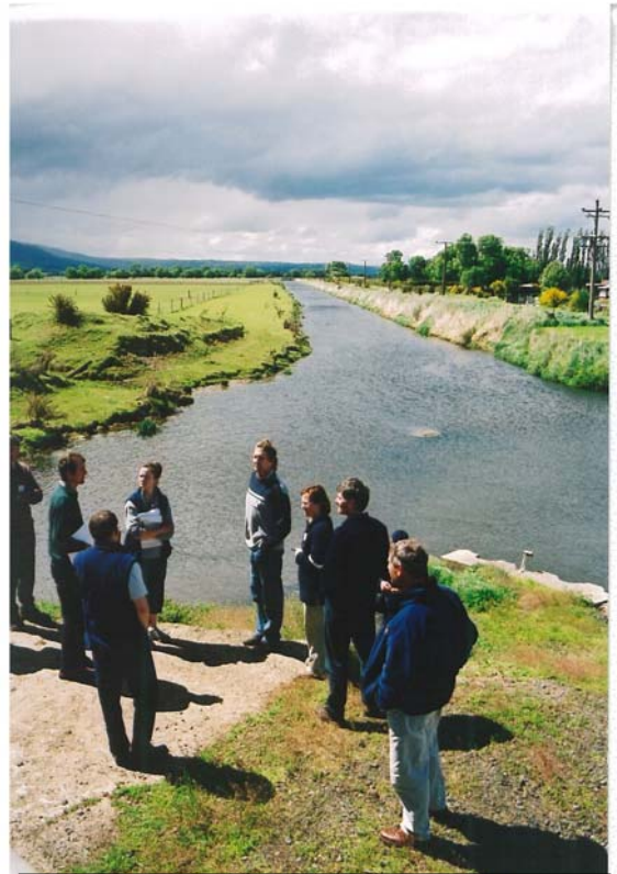
Photo 2: A view of the Main Drain before it discharges by pump into Lake Wainori Drains Workshon
