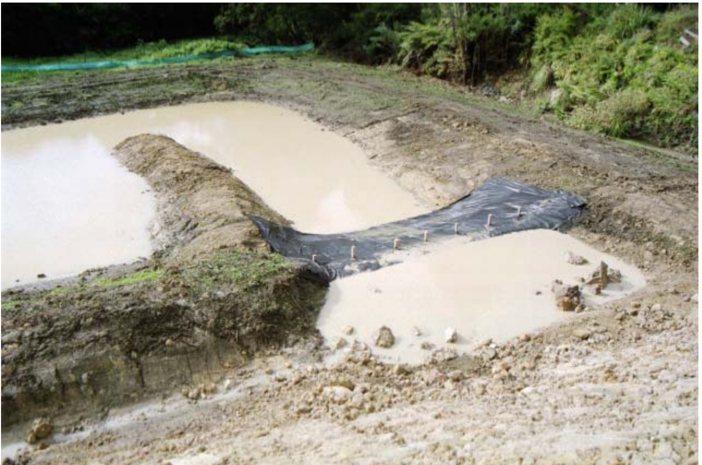
Sediment Control pond - Auckland
