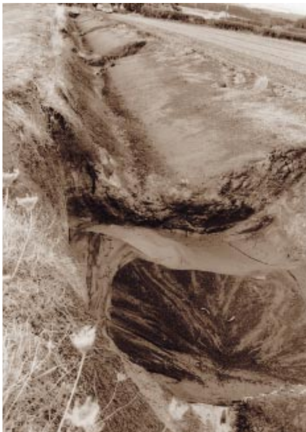
Silt traps. Photo: Franklin Sustainability Project.
