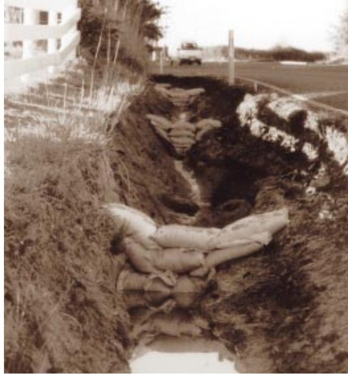
Sandbags used to control drain velocity.
