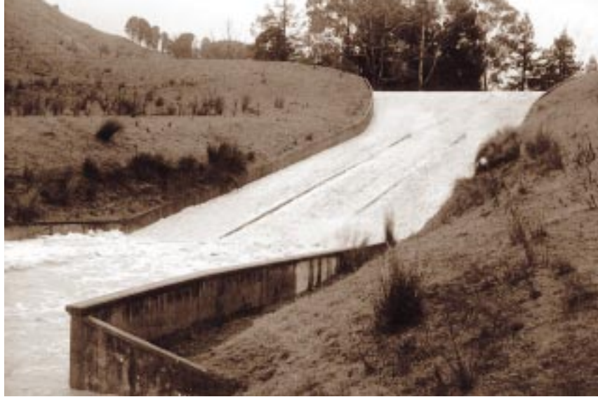
Concrete drop structure – spillway over dam.
