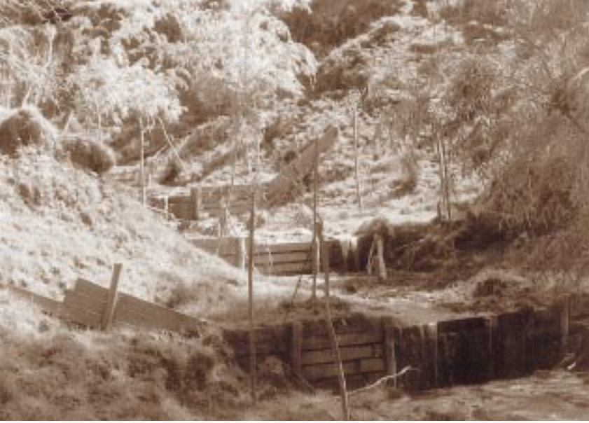
Timber debris dams. Photo: Gisborne DC.
